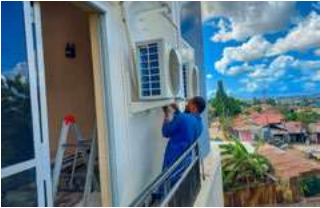
Installing an outdoor unit on a house
